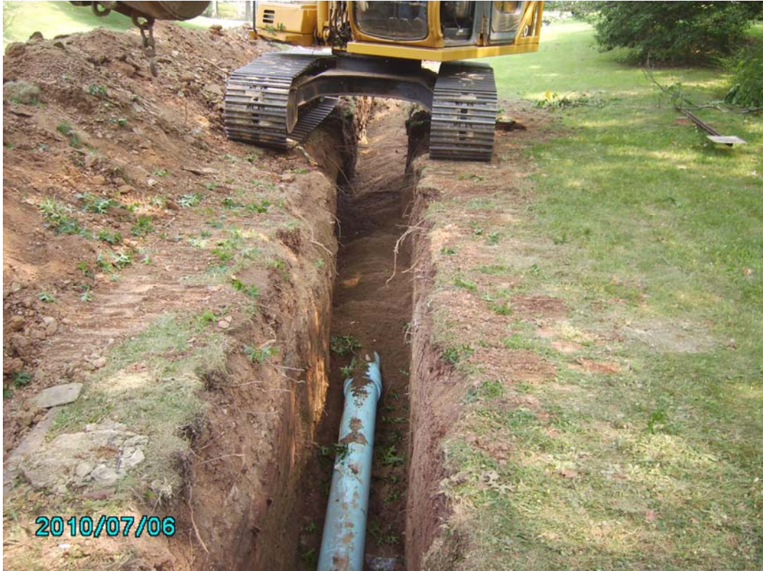
Install New 8" PVC Waterline
