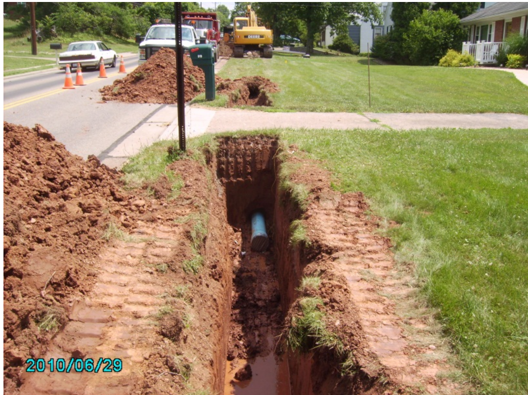
Driveway's Bored Where Possible to Reduce Inconvenience to Homeowners
