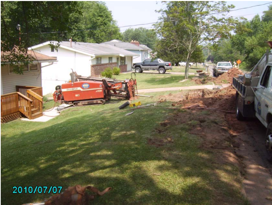
Directional Drill Service Lines
