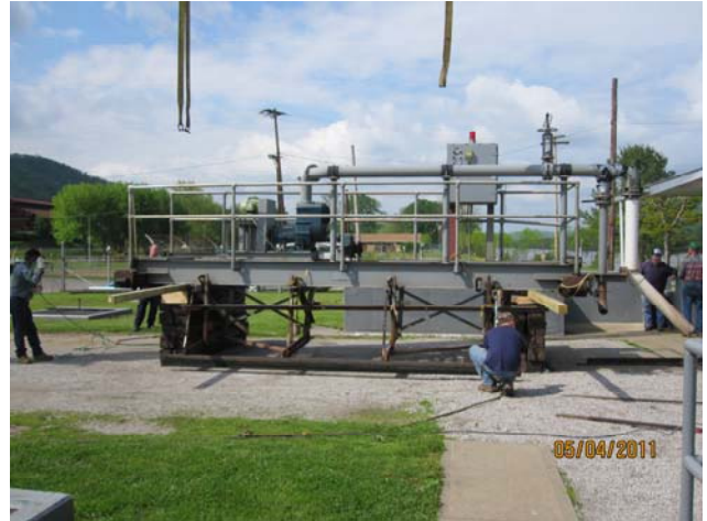
Bridge ready to be rebuilt onsite
