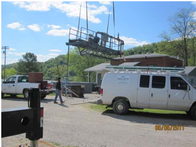
Rebuilt bridge lifted back onto clarifier
