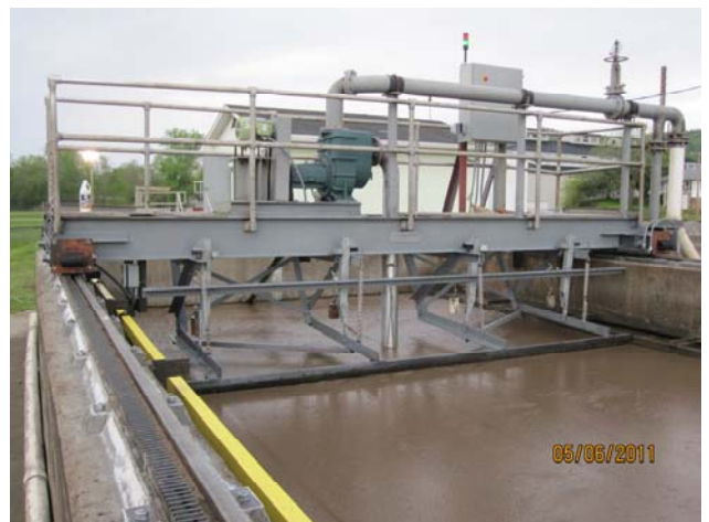
Clarifier Bridge back in service
