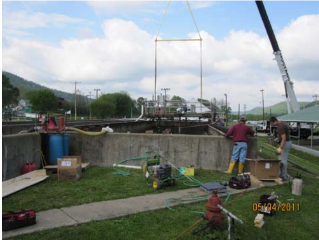
Bridge ready to be removed for repair
