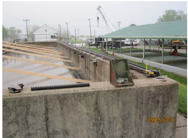
New Rail & Drive Rack were installed
